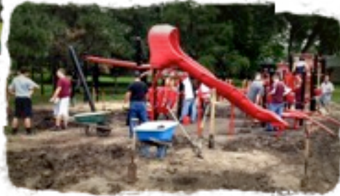
Volunteers & staff helping construct the new elementary play structure.
